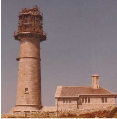
Old Light with scaffold.
