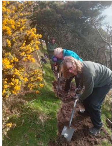
Hard at work levelling the path leading to the Ugly.
