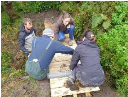
Rebuilding the bridge next to the Casbah. Photo by Jane Elliott
