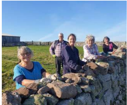
Dry stone walling near the Lambing Shed. Photo by Jane Elliott
