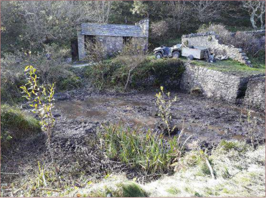
Millcombe Pond post-clearance. Photo by Bob Bagatti
