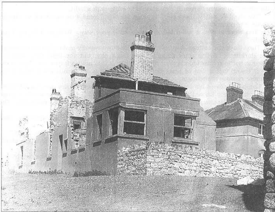
Above: From left to right, the Coastguard Cottages and Signals
