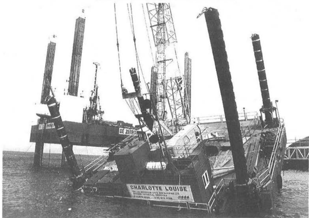
The collapse of the construction platform Charlotte Louise
