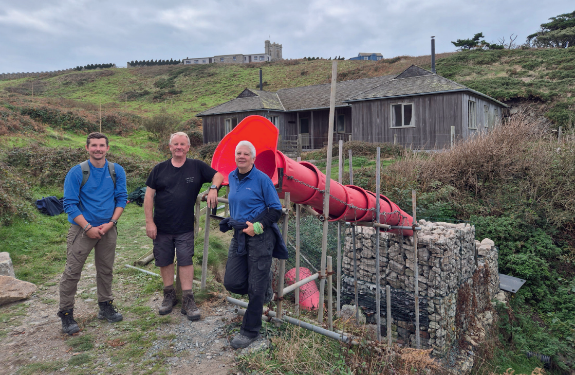
▲ Roger and Zdena at Bramble's Gabion Baskets (photo: Hilary Winsor)
