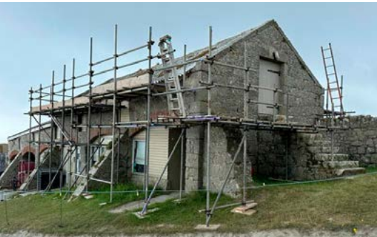
▲ Scaffolding enshrouding the General Store during renovation work (photo: Derek Green).
