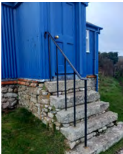
▲ The new forged rails on the steps up to the Old School (photo: Derek Green).
